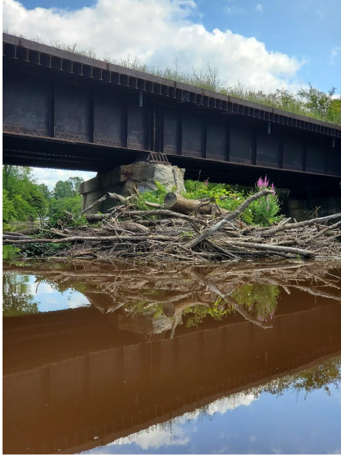
Figure 30. Large Obstruction forming at coordinates 42.945625, -79.039540 under the railway bridge.
